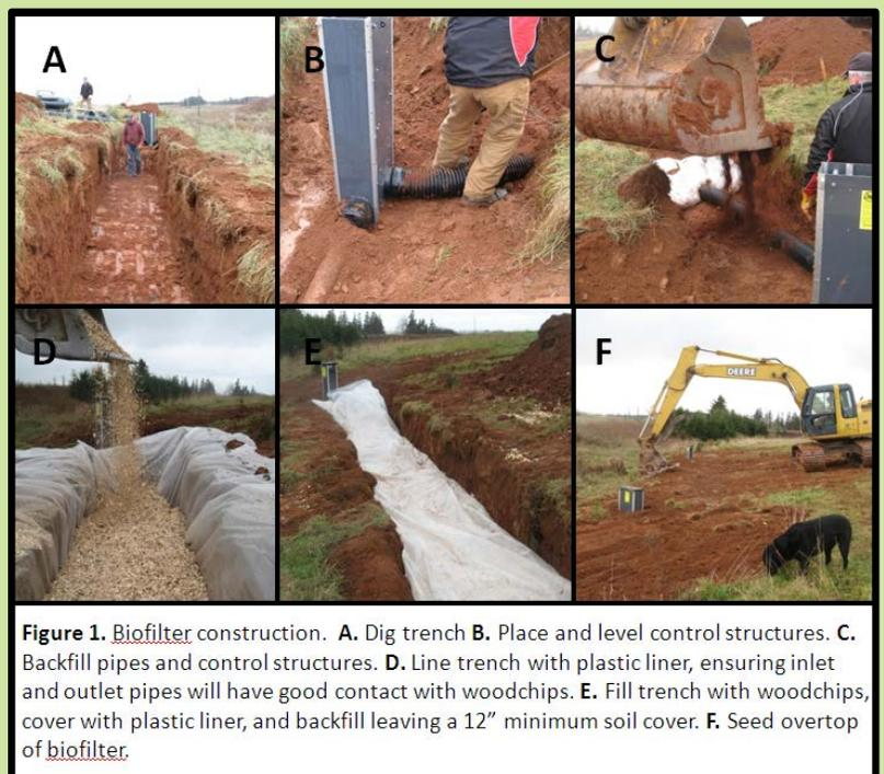
**Figure 1.** Biofilter construction. A. Dig trench B. Place and level control structures. C. Backfill pipes and control structures. D. Line trench with plastic liner, ensuring inlet and outlet pipes will have good contact with woodchips. E. Fill trench with woodchips, cover with plastic liner, and backfill leaving a 12" minimum soil cover. F. Seed overtop of biofilter.
